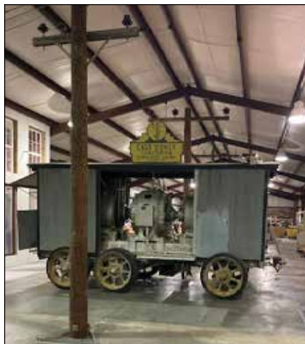
1920 Westinghouse Portable Substation.
