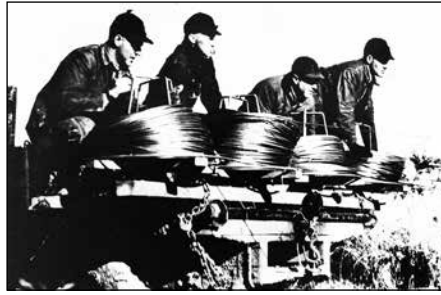
The famous photo of the four horsemen operating the payout reels of overhead conductors that were being installed on a rural line extension.
