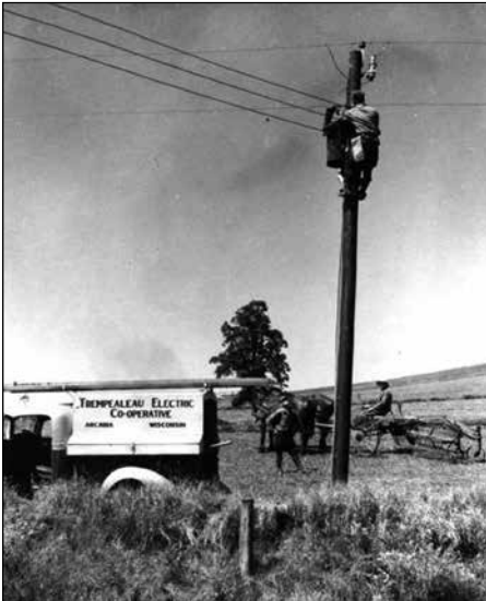
Showing a Cooperative lineman connecting a service to a farmer's ranch.
